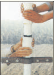
Always hold the coupler of pipe by hand or wrench during fitting of pipe so that coupler does not get turned.
