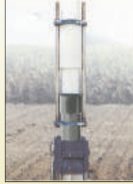
Fit male square threads of X-illant column pipe with female thread of pump guard / adaptor.
