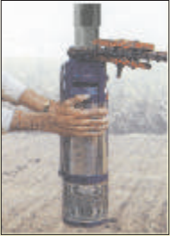
Fit male thread of C.I. adaptor with female threads of submersible pump using chain wrench.
